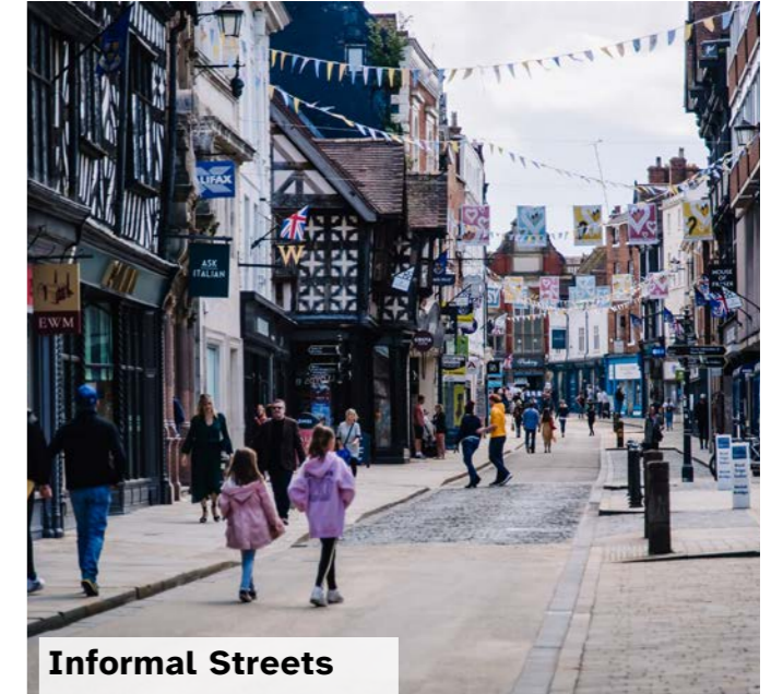
Figure 15 Informal Streets accommodate traffic, but at slower speeds, and offer increased space for pedestrians and cyclists. Formal traffic controls are absent or reduced. There is a footway and carriageway, but typically there is less differentiation between them such that it is typically less than in a conventional street.
