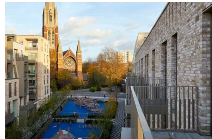
Figure 73 Balconies can project up to 2m and should be fully integrated in the design of the building.
