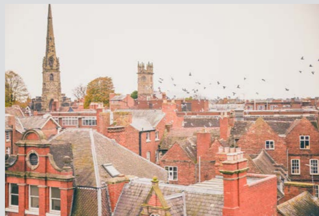
Figure 12 View of Shrewsbury's roofscape with St Alkmund's Church spire and St Julian tower.
