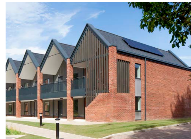
Figure 74 Orientating roofs to incorporate PVs. Radbrook Village, Shrewsbury. Photo credit AHR Architects.
