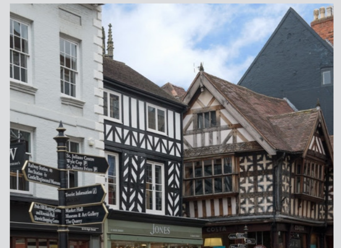
Figure 10 Variety of buildings along High Street.
