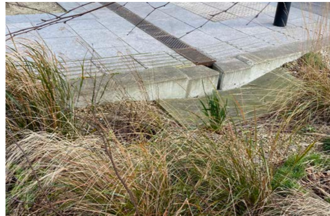
Figure 44 Sustainable Urban Drainage including rain gardens, within the design of public realm.
